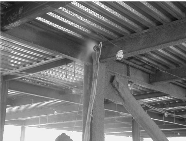
The thickness, bond strength and density of the fireproofing material must be tested. Since the required fireproofing thickness varies depending on the size of a steel beam or column, the inspector needs to have a copy of the approved thickness schedule in order to perform the testing. The code
